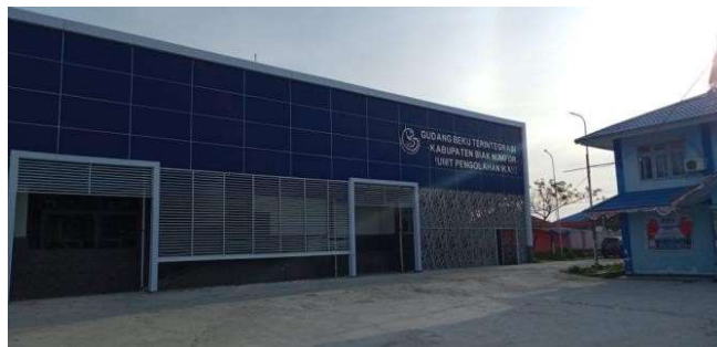
Figure 1. Cold Storage In Binyeri Village
